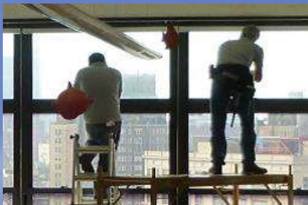
SerraGlaze Daylight Redirecting Film is installed in the upper portion of the window.
